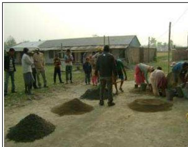
Figure 11 Measuring sand and soil proportion at Morang district
