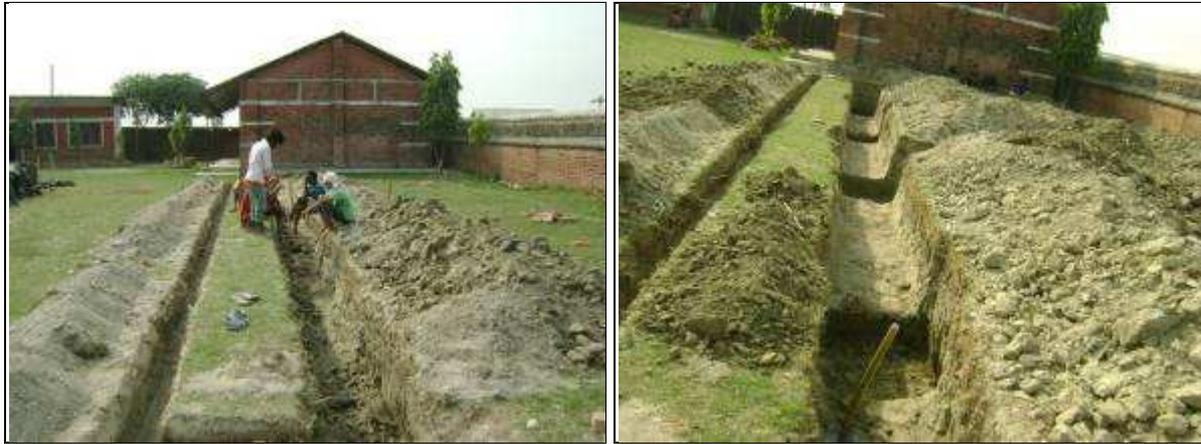
Figure 16 excavation of foundation at Morang district
