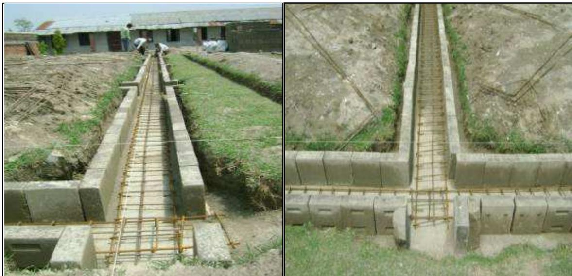
Figure 18 Framing and arranging reinforcement for concreting of foundation ring beam
