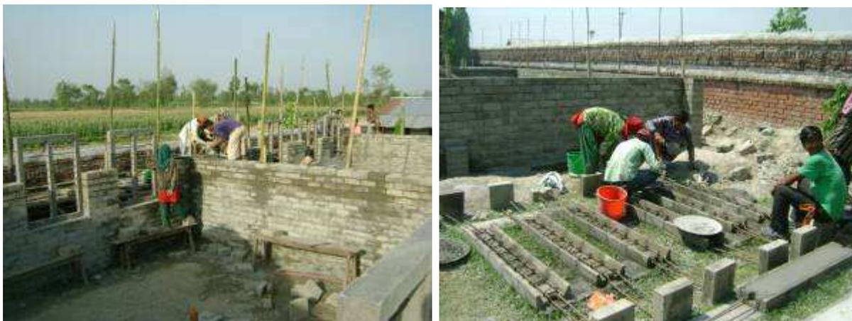
Figure 28 block work at corner tie and preparation of lintel
