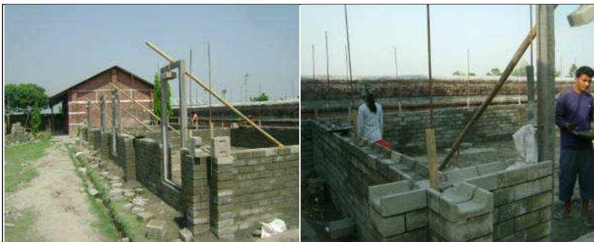
Figure 25 sixth layer from plinth level and arrangement of U-Block for sill ring beam
