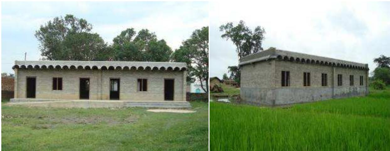
Figure 30 Ferro Cement Channel roofing system at bake district
