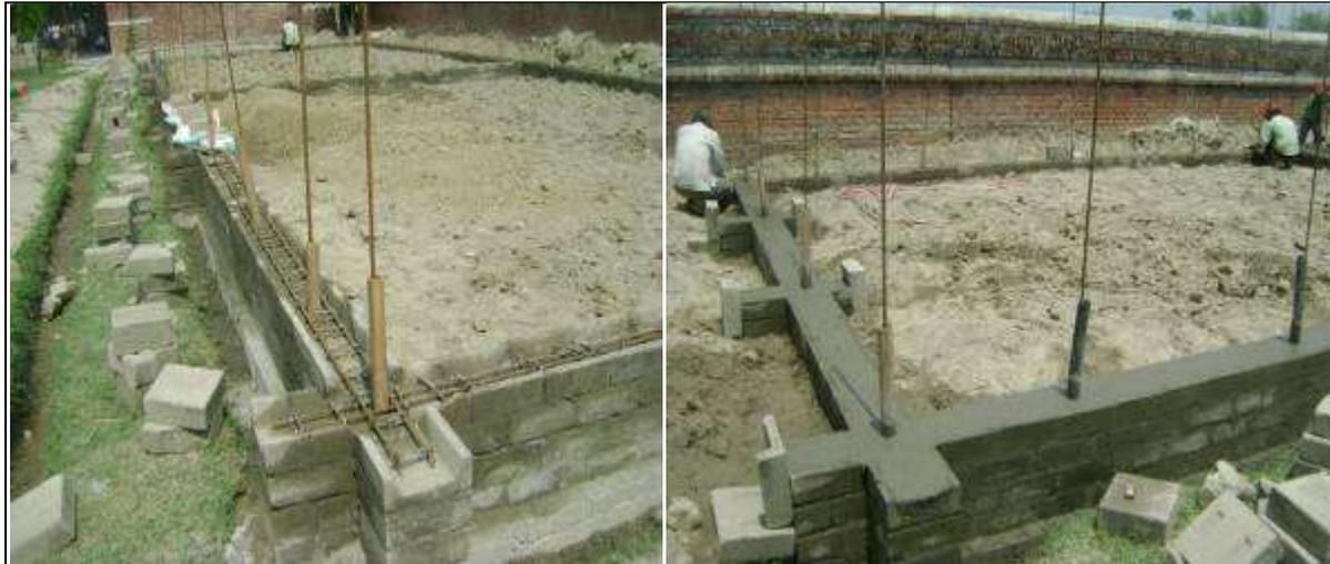
Figure 23 arrangement of reinforcement and concreting of plinth ring beam
